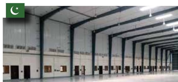
Air Force hangar Pakistan | HANGAR
